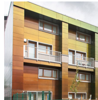
Ernley Close, Manchester (Source: 2e Architects)
