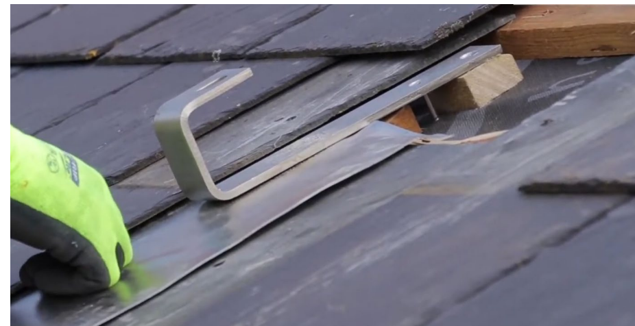
Products and processes have been specifically developed to securely fit panels to existing roofs. Example shows a stainless steel roof hook being mounted to a slate roof. (Source: Schletter installation video)
